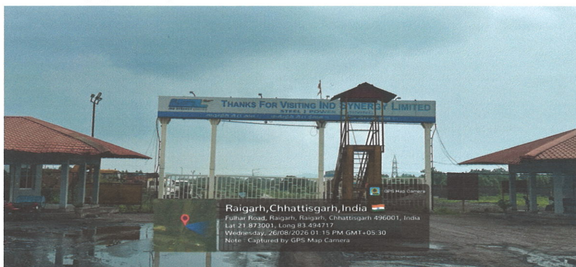
Figure – 4, Entry Gate for Material
